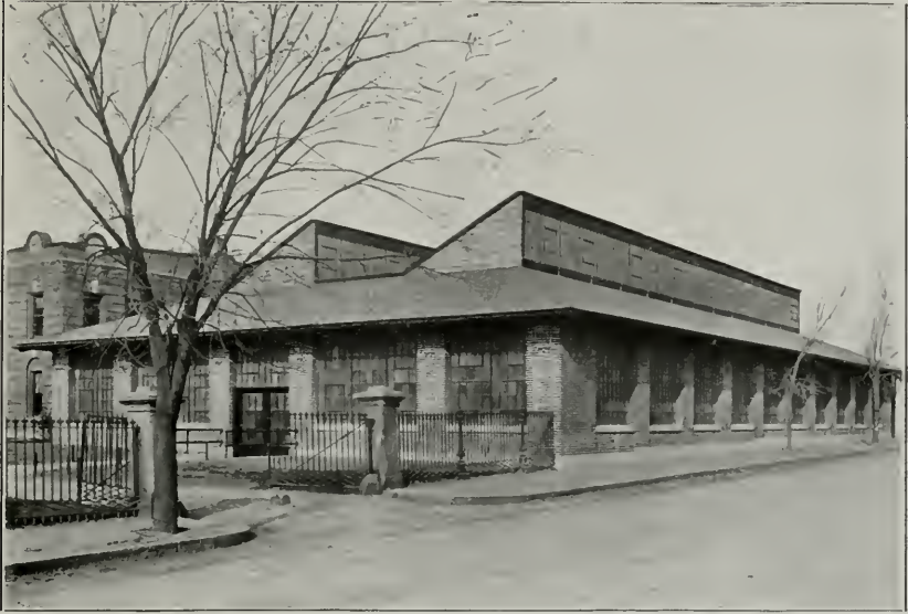
THE NEW PRESS-ROOM BUILDING
